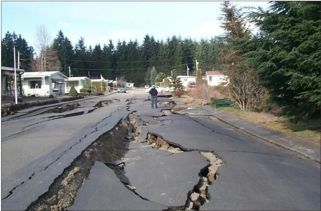
Road damage from the 2001 Nisqually Earthquake in Thurston County, Washington.
