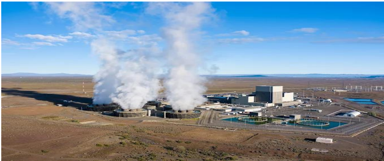
Columbia Generating Station, located just north of Richland WA
