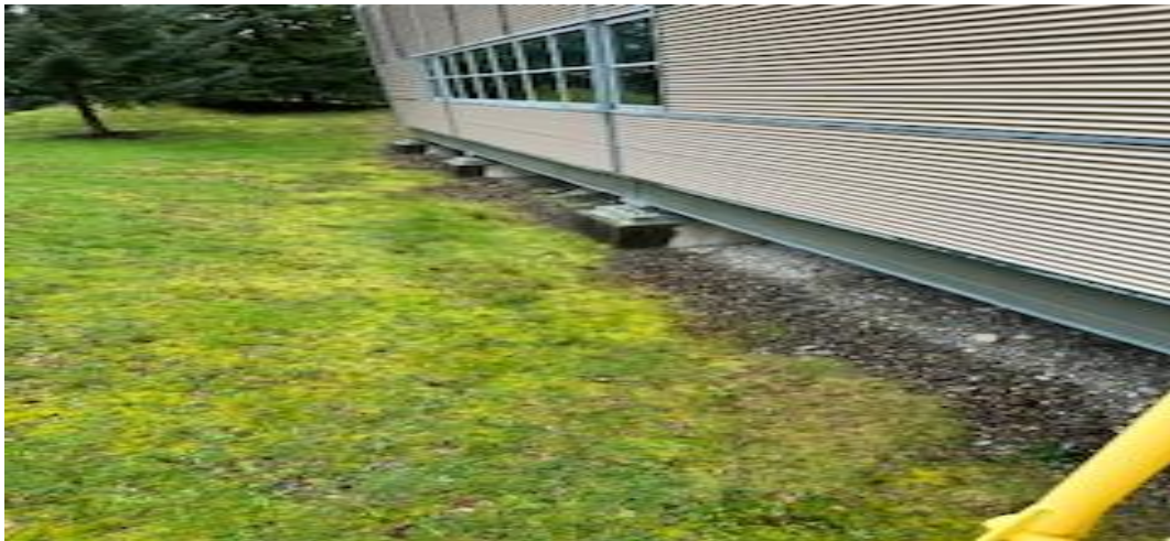
Side view of Washington EOC building showing steel-braced resting on framed base isolation foundation. Photo courtesy of Craig Johnson (NG7N).
