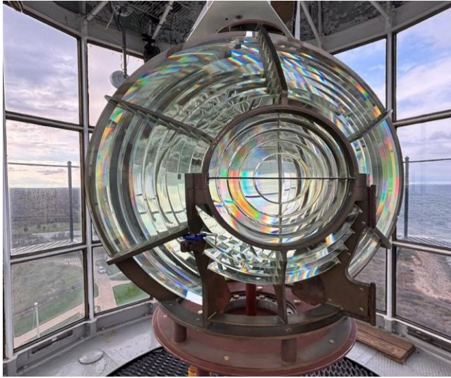
A Fresnel Lens in the Montauk Point, Long Island, NY lighthouse.
